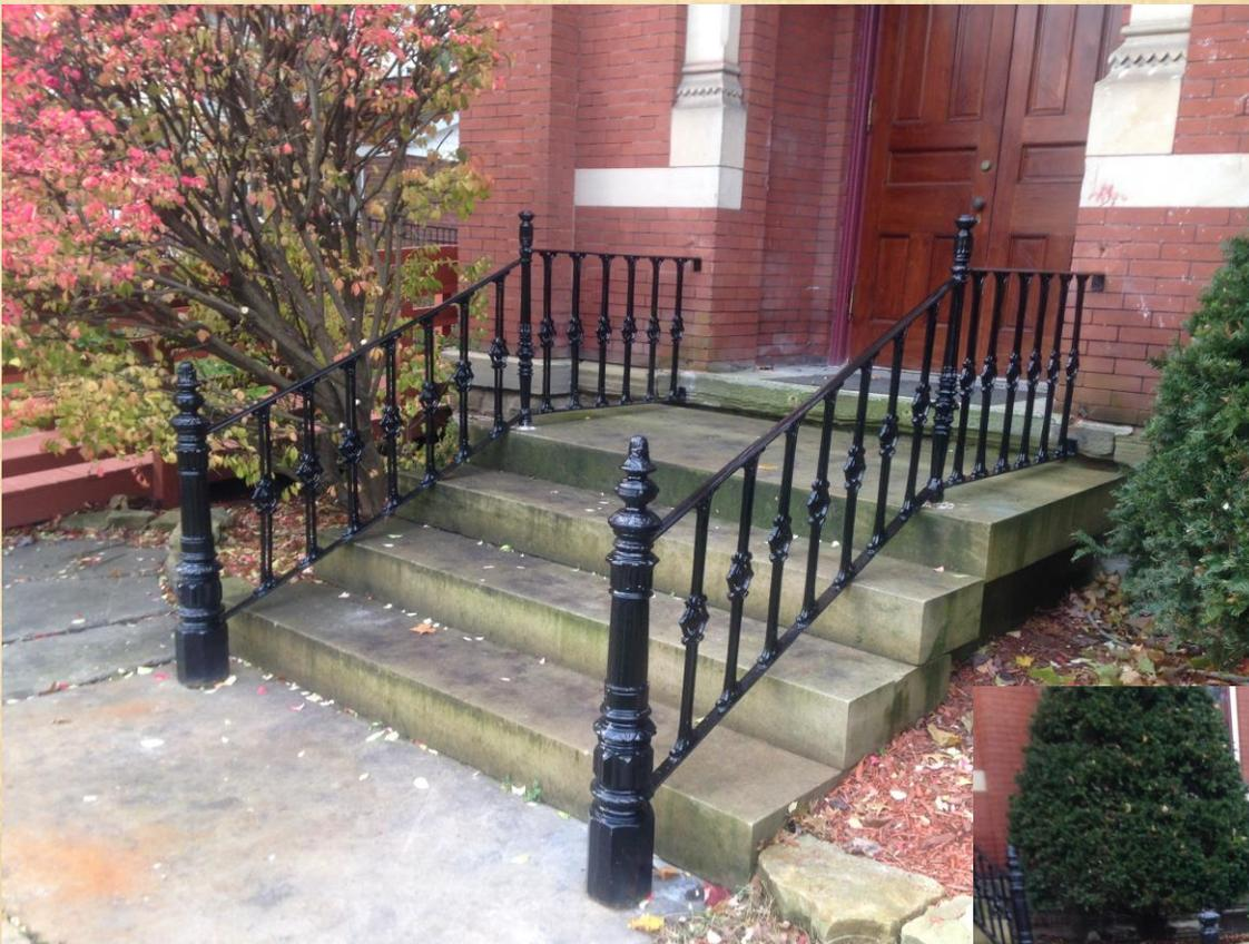
The summer of 2017 saw the replacement of the badly-deteriorated front steps of our headquarters building with sandstone slabs in concordance with the original construction.
